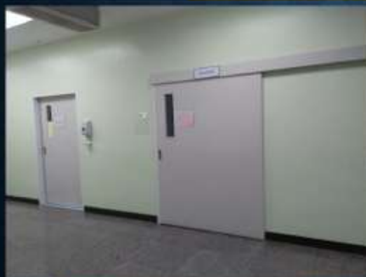
Negative pressure room
